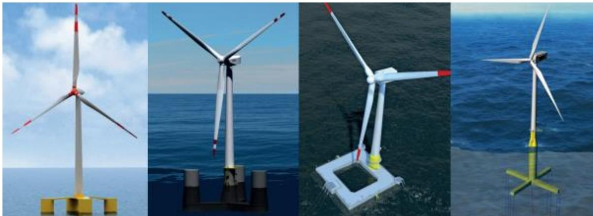
**Figure 1: Semi-submersible steel design, Semi-submersible concrete design; Barge concrete design, TLP steel design**
