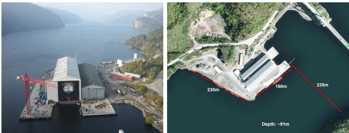
Figure 17. Details of the Kvina yard at Kvinesdal proposed for WTG installation (concrete).
